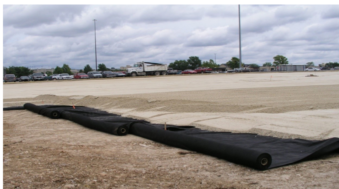
Figure 15 - Nonwoven deployed on subgrade
