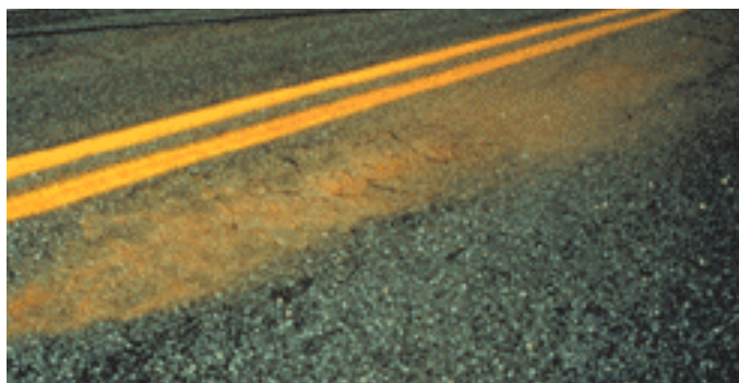
Figure 1 - Subgrade pumping
