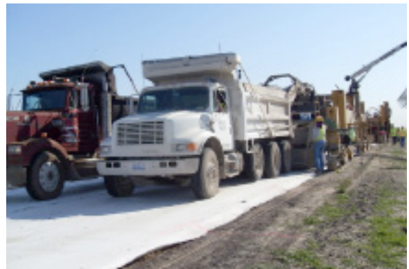
Figure 1 - Haul Trucks Unloading Concrete across Reflectex
