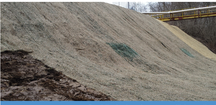
INSTALLATION Rapidly deployed system utilizing soil, seed and ECB to establish vegetation
