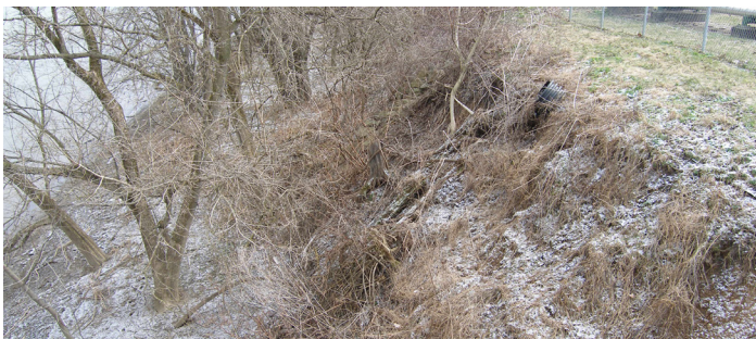
PROBLEM Property loss and dangerous drop off
