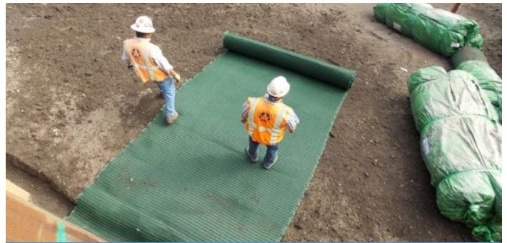
SOLUTION ARMORMAX® 75 shown along the bank to the water's edge
