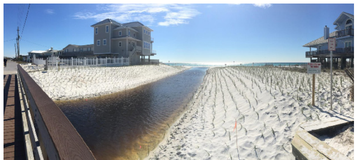
PERFORMANCE The vegetated slopes of the outfall withstood extreme conditions from Hurricane Michael
