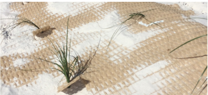
INSTALLATION More than 2,000 sea oats were planted into the ARMORMAX system
