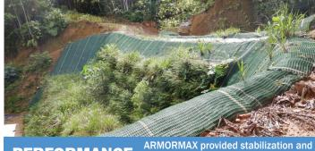
PERFORMANCE ARMORMAX provided stabilization and permanent erosion protection
