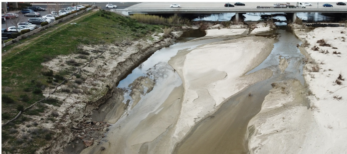
PROBLEM Erosion and scour of Murrieta Creek banks due to flooding events
