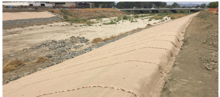
SOLUTION ARMORMAX ® 75 was chosen as the solution for Phase 2A as it provides significant time and cost savings as opposed to hard armoring solutions like concrete
