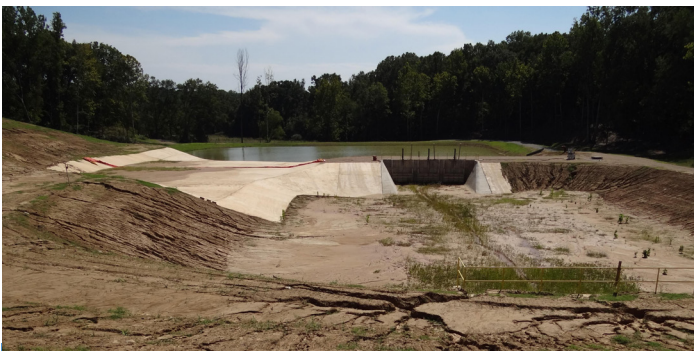
PROBLEM Extreme erosion due to heavy rainfall
