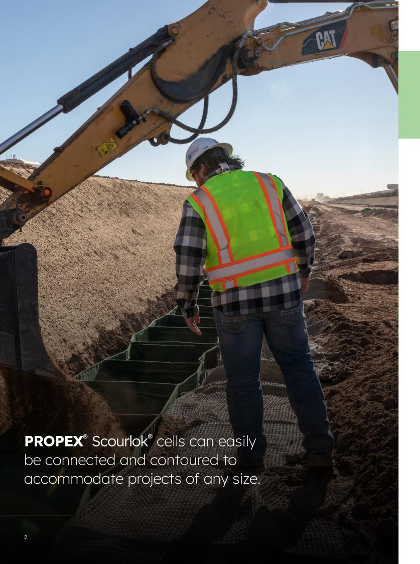
PROPEX Scourlok is a robust Engineered Bank Stabilization system designed to resist extreme hydraulic stresses and protect shorelines while promoting vegetation.
