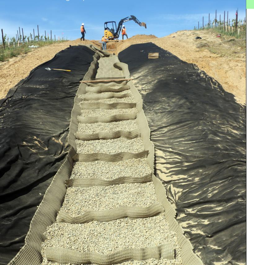
The system utilizes the durability and erosion resistance of PROPEX Pyramat 75 High Performance Turf Reinforcement Mat (HPTRM) to construct a geosynthetic/soil/rock composite for protection of channels, slopes, and spillways.
