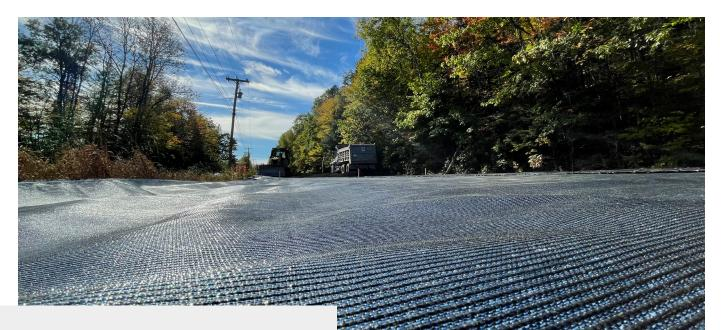
MIRAFI H<sub>2</sub>R*i* has unique hygroscopic wicking yarns that provide enhanced drainage along the plane of the geosynthetic. This leads to a unique ability to remove water from roadways and other structures in unsaturated conditions.
