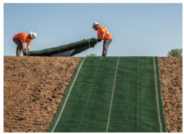
**HPTRM Laydown:** Unroll the HPTRM on the prepared soil ensuring material has intimate contact with the soil.
