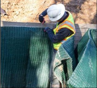
12. Repeat Steps 1 through 11 for each subsequent unit. Incorporate a setback with unit to provide the desired overall slope angle.
