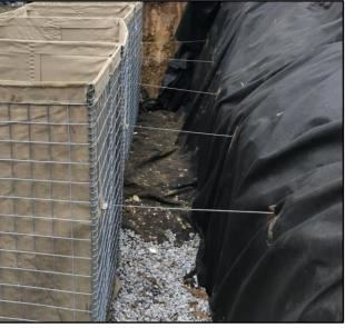
7. Place a 6 in (15 cm) thick fill material approved by the Engineer within the units. Check and adjust the units to ensure a level placement. If joining the units together in series, do not fill the end cell more than 6 in (15 cm) prior to joining units.
