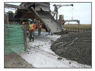
As concrete interlayers, REFLECTEX and GEOTEX 1341NH provide cushion and drainage between an existing pavement layer and a concrete overlay. They also prevent bonding between the new overlay and the existing pavement below.
