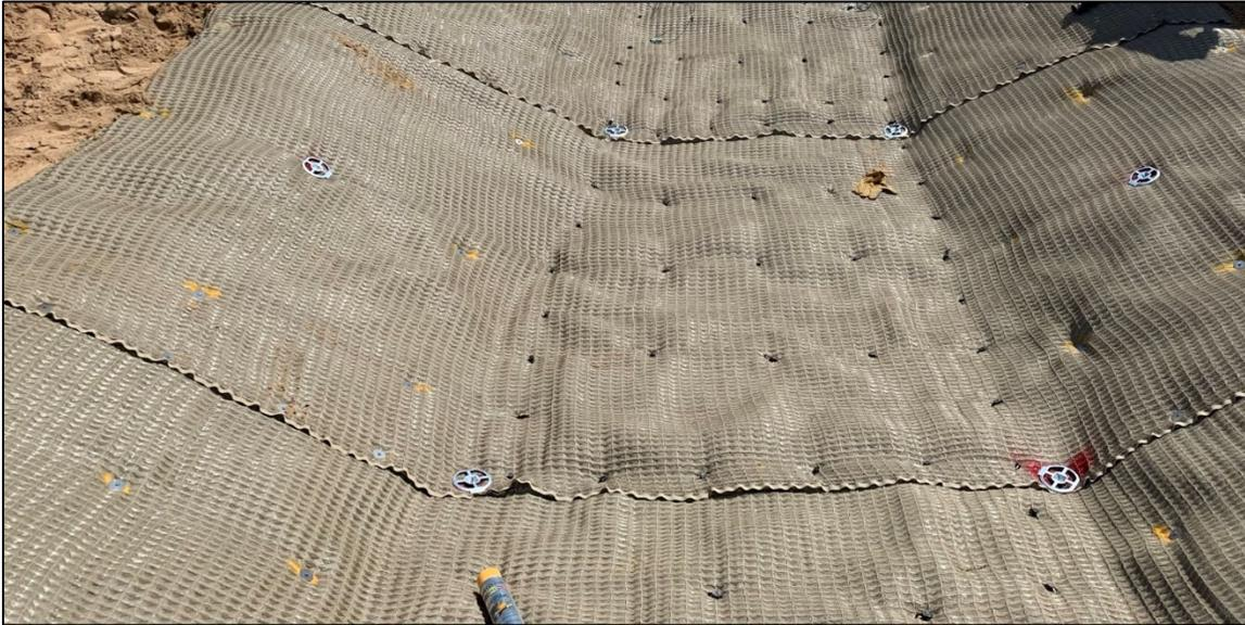
**Figure 6- Overview of Overlap and Synthetic stake spacing**
