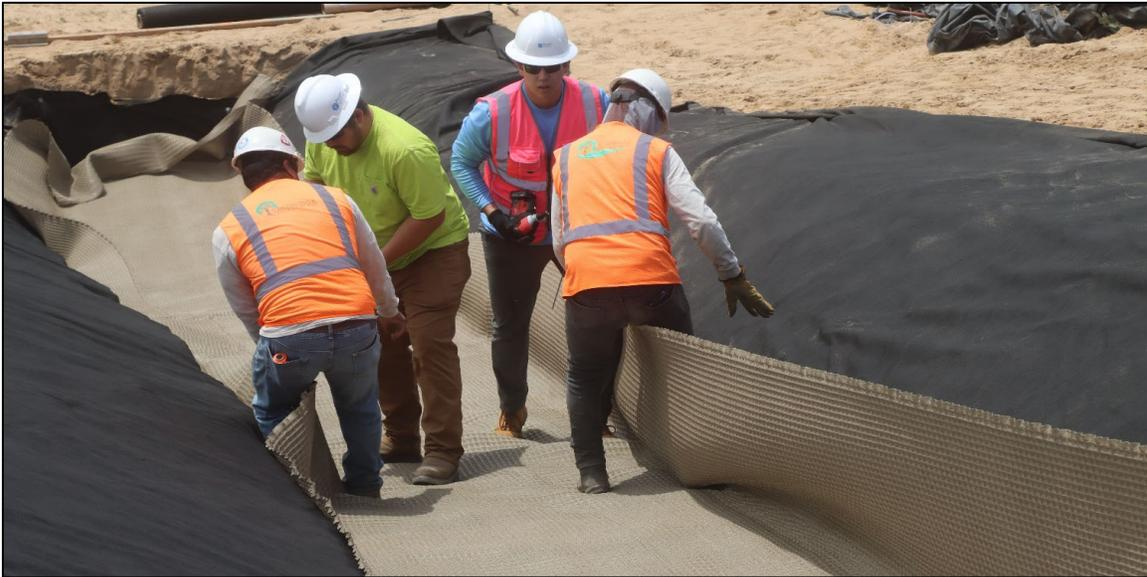
**Figure 2- HPTRM placement in bottom of excavation**
