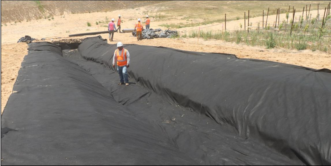
**Figure 1- Geotextile placement in excavation**
